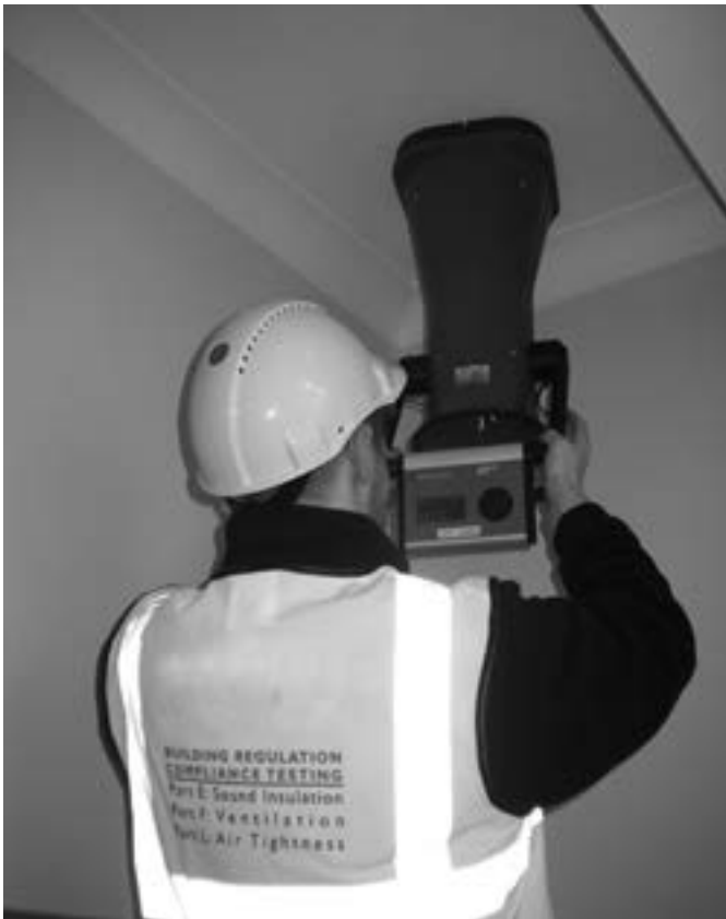
Figure 2.37 Flow hood (reproduced courtesy of BSRIA Compliance)
